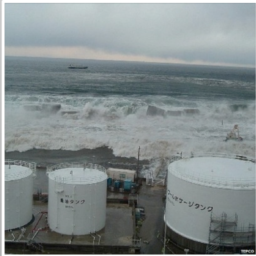
Fukushima Daiichi Nuclear Power Plant and Reactor Unit Damage
